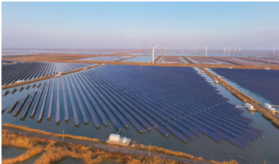
Xiangshui, Jiangsu 170MW photovoltaic agriculture project
