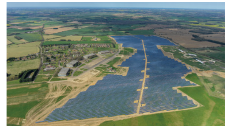
Norfolk, Britain 50MW ground-mounted power station project
