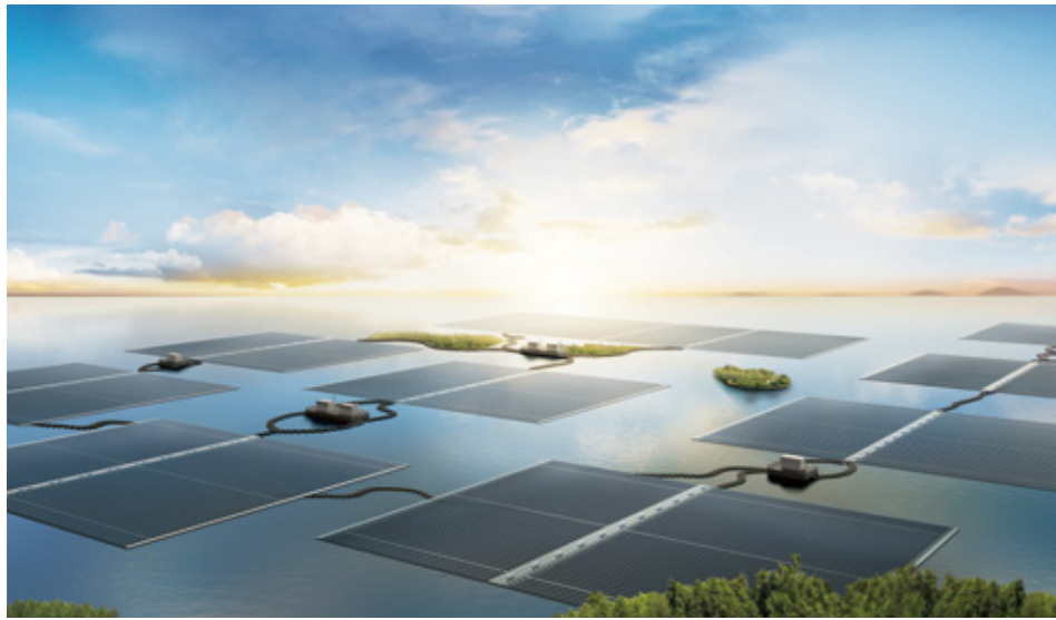
Lianghuai, Anhui 170MW floating project
