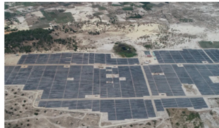
Phong Phu, Vietnam 42MW ground-mounted power station project
