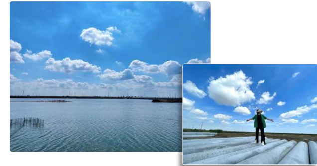
Hebei Nandagang 70MW Fisheryvoltaic Complementary Project
